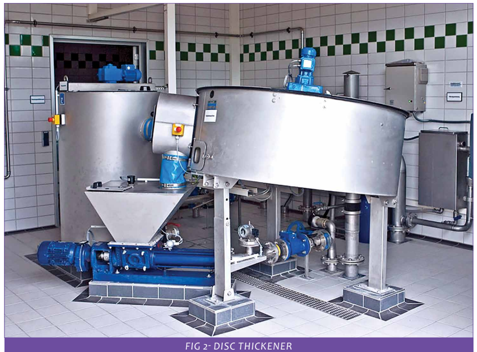
FIG 2- DISC THICKENER
